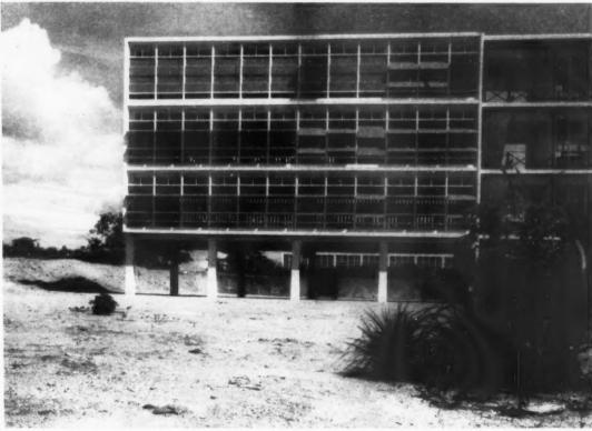
windows glazed with non-actinic glass and movable through 135°. Below the clerestory are continuous rows of pressed steel doors containing glazed panels and openings of small adjustable louvres. The entire sides of the building can therefore be opened up to catch
