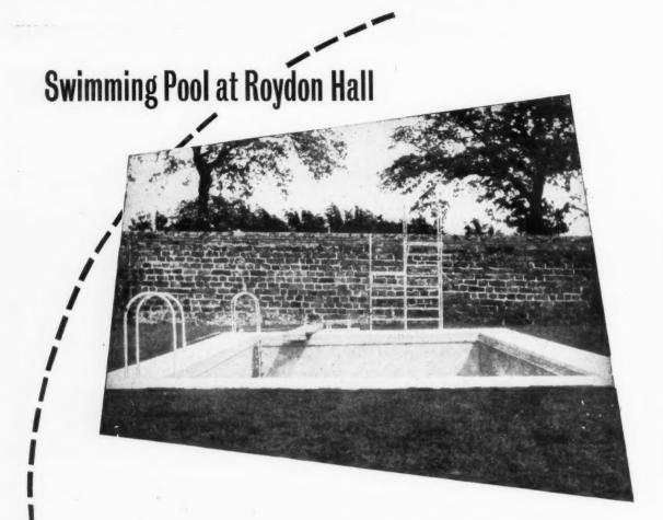
In the lovely grounds at Roydon Hall, Norfolk, a swimming pool has been constructed for John Alley, Esq., J.P. The pool is 34 ft. long and 20 ft. wide, one end being 3 ft. 6 ins. deep increasing in the middle to 8 ft. and decreasing at the other end to 6 ft.
