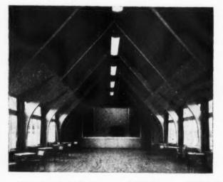
Interior of one wing showing buttress type laminated timber beams in Sir Herman Lebus Sports Pavilion at Tottenham. Designed, manufactured and erected by Kingston (Architectural Craftsmen) Ltd.
