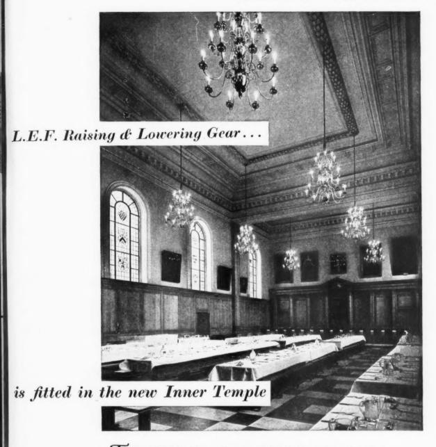
he beautiful Hall of the new Inner Temple is lighted by ten heavy chandeliers weighing about 2 cwt. each. They are brought down to floor level for convenient maintenance by means of L.E.F. Raising and Lowering Gear.
