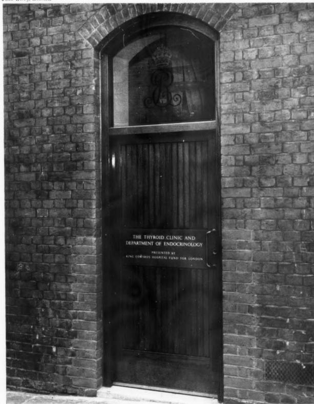
This external door is fixed in an existing door opening. The name-plate is stove-enamelled mild steel. The cipher in the fanlight is etched on  $\frac{1}{2}$ -in. plate glass.
