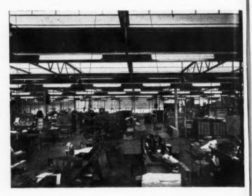
working plane. The use of such two-side lighting also has the advantage of avoiding shadows that are created with one-side systems such as the old-fashioned north light roof truss, which result in restrictions on production layouts, or if the lighting is ignored, poor working conditions with operators working in shadows. The detailing of the monitors is similar to those on the prototype factory (see Working Detail, AJ, April 7, 1955) and a detail section is illustrated on page 354.
