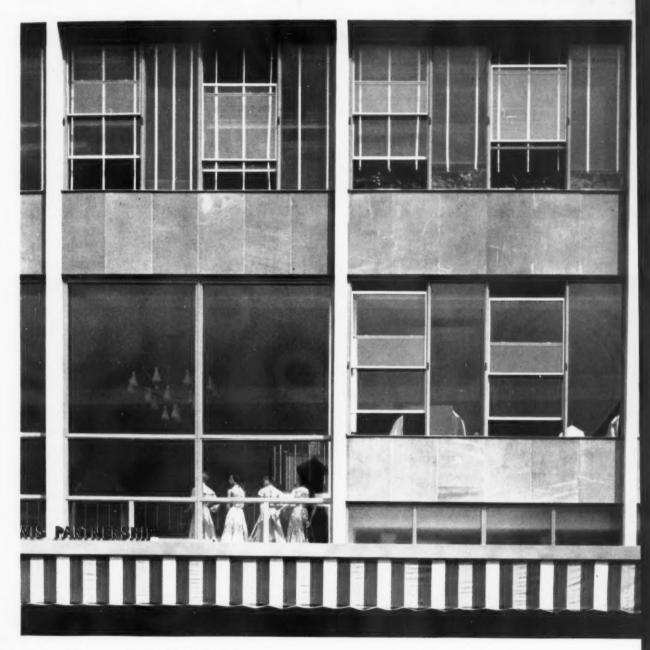
The building is designed to take additional storeys at a later date, as will be seen from the drawing where prorision for the cramps of future slate facing panels is made behind the Portland stone fascia.
