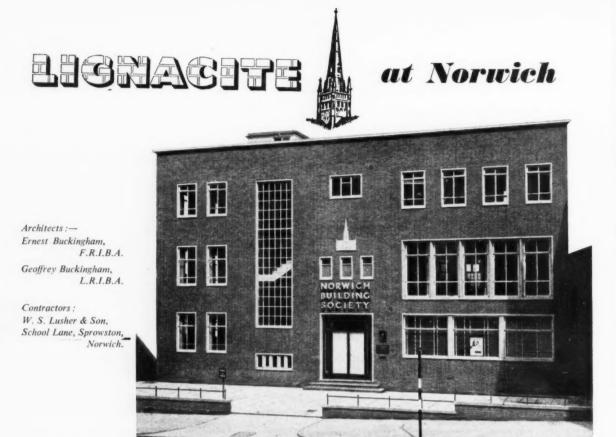
THE Norwich Building Society new head offices at Norwich, where 850 yards super of 4in. thick Lignacite Lightweight Concrete Blocks were used in the construction of the internal walls. This is yet another of the wide variety of buildings, public or private, large or small, for which Lignacite Blocks are proving their superiority.
