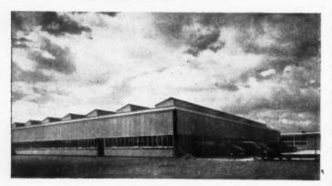
Above (viewpoint 7): the standard cladding runs round the north-west and east sides of the production area. As with the prototype, the corner stanchions are in the form of welded steel boxes, exposed externally and painted black, thus avoiding the need for specials with the patent glazing or the asbestos sheeting. Apart from this steelwork and the plinth formed by the exposed edge of the ground beams,
