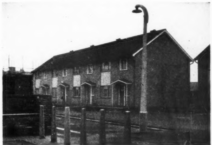
The light post and rail of the access galleries of the West Ham flats, above, show a neat way of handling the problem of external access. The rendered panels between the porches emphasise the individual house in this terrace, below. Bottom, two-storey flats.
