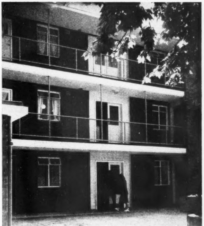
The light post and rail of the access galleries of the West Ham flats, above, show a neat way of handling the problem of external access. The rendered panels between the porches emphasise the individual house in this terrace, below. Bottom, two-storey flats.
