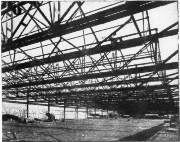
① New factory building for Messrs. William Cooke & Co. Ltd. of Rotherham. 300 ft. x 120 ft. span.
