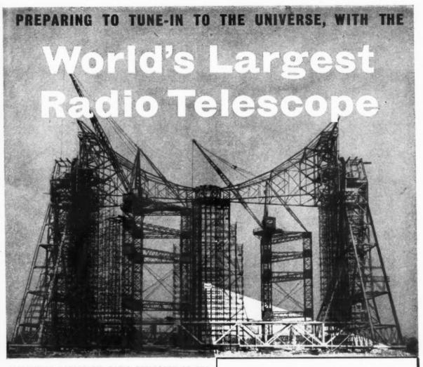
ALTAZIMUTH PARABOLOID RADIO REFLECTOR AT THE JODRELL BANK SITE, BUILT FOR MANCHESTER UNIVERSITY AND THE DEPARTMENT OF SCIENTIFIC & INDUSTRIAL RESEARCH. CONSULTING ENGINEERS: HUSBAND & CO., SHEFFIELD. STEELWORK CONTRACTORS: UNITED STEEL STRUCTURAL CO. LTD.
