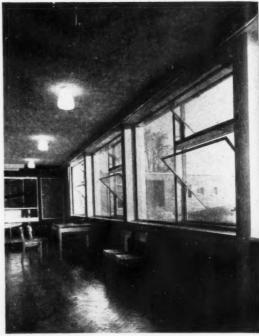
tubular sections with handrail and bookshelf in polished mahogany. Finishes: walls plastered, with painted finish ceiling, vermiculite plaster; floor, wood block.
