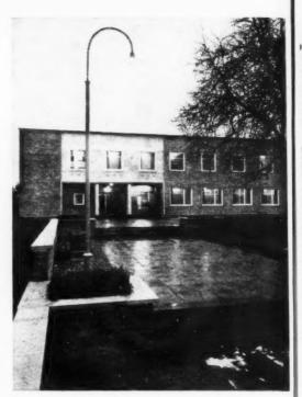
Viewpoint 2: the public entrance approach and steps and the terrace to the entrance front are paved with special concrete slabs. Brick flower boxes with artificial stone copings are placed either side of the two short flights of steps. On one side of the entrance approach there is cobblestone paving between the flower boxes; inserted in these are plain concrete paving slabs, which carry the wooden seats.
