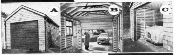
(A) Counterbalanced by powerful springs, the door slides—not tilts—upwards when unlocked.
