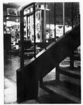
Above left: another view of the staircase to the basement. The non-slip treatment of the suspended treads is shown in the detail, left, Above: the main staircase to all floors lies on the north side of the block. It is cleanly detailed with precast terrazzo treads and in situ coved corners for easy maintenance. The simple but decorative handrail is firm and rigid without appearing heavy. Coloured tile panels identify floor levels.
