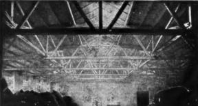
Scientifically constructed, with pre-formed bows of laminated wood.
