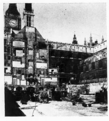
— with foundations well below Thames high water level, the House of Commons was rebuilt in 1946 to last for centuries, and was therefore protected with *mastic asphalte* laid by a member company of the Asphalte Council.
