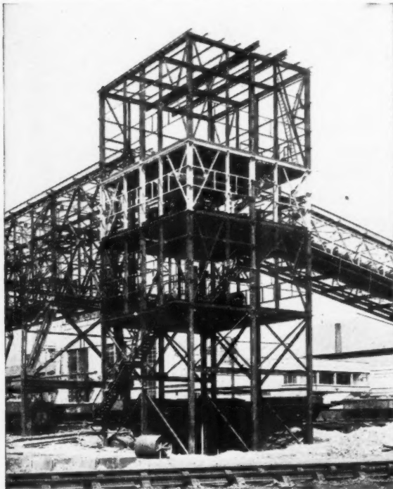
Steelwork for Raw Materials Handling Plant, installed by Mitchell Engineering Ltd., at the gigantic new Works of the Steel Company of Wales at Margam.
