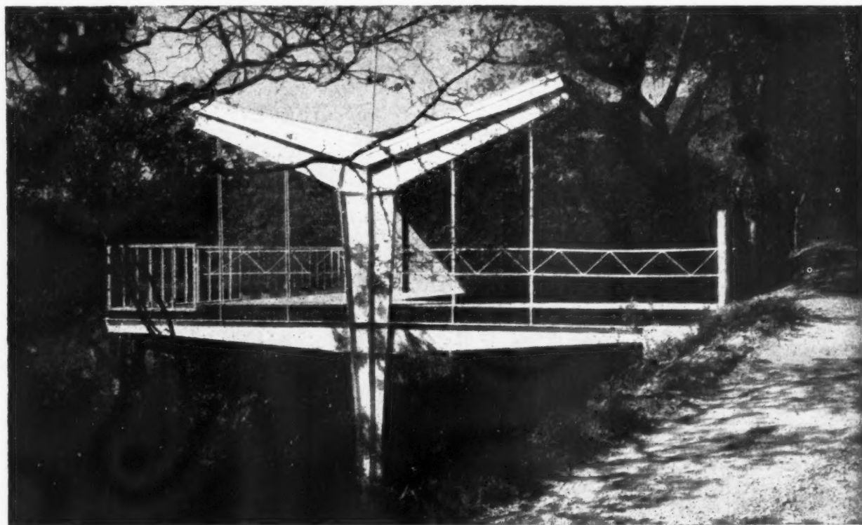
Fig. 8: the structure of the Corns House consists of standard steel three-hinged frame members placed back to back. The only foundations required on a 45-deg. sloping site were a row of five pads. The external walls are a sandwich of aluminium sheet, glass fibre and plywood, 1½ in. thick.
