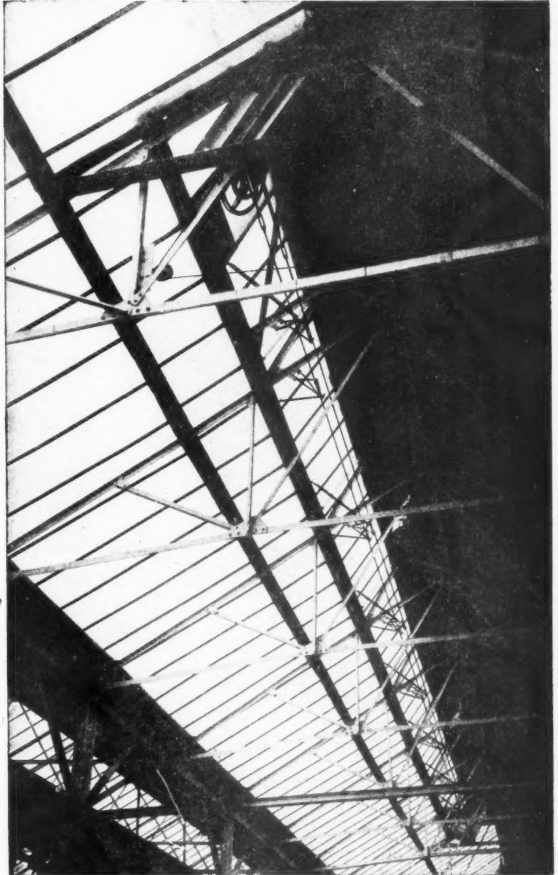
The illustration shows One set of Electrically operated Twin Tension Rod Gear with Counter-Balance Unit operating one continuous opening light, 74' 0" long x 5' 0" deep. Note the Spiral Balance Wheel fitted at the end sprocket.
