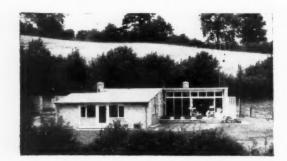
This single-storey, three-bedroom house, built on a sloping site, was designed by the architect for his own use. Oil-fired under-floor heating with independent control of the heat supply to different parts of the house, has been used. The L-shaped plan encloses a terrace overlooking the Wiltshire Downs. The final cost is estimated at about £6,250, including external work.
