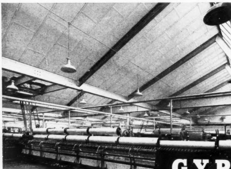
Insulating Gypstele Ceiling erected in the Spinning Card Room at John Barnes & Sons Ltd., Tennyson Road Mill, Preston.
