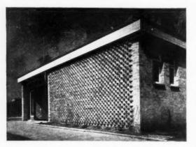
Viewpoint 8: a detail view of the fish and chip shop. The entrance on the left comprises a fully-glazed door adjacent to a large plate glass window. The assertive brickwork texture is achieved with projected headers laid diagonally.
