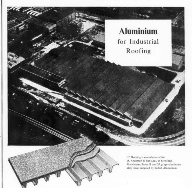
Illustrated is the new extension at Warrington for the Thames Board Mills Ltd., one of the largest manufacturers of board for packaging and fibreboard cases in the world. Its vast roof, consisting of a main area covering 250,000 sq. ft, is entirely covered with Anderson Aluminium 'E' Decking.
