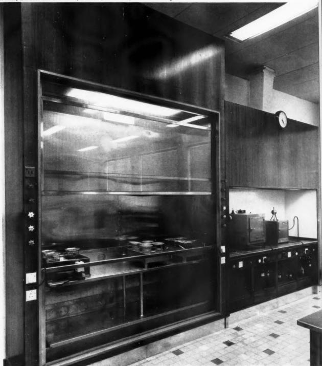
The service connections in the building are designed to permit fume cupboards to be connected at 10 ft. intervals, as required. The fume cupboards are therefore demountable and are designed to permit easy connection to the services. They are also provided with a double work-top: a removable top at normal bench height and a low level work-top to permit the use of tall equipment.
