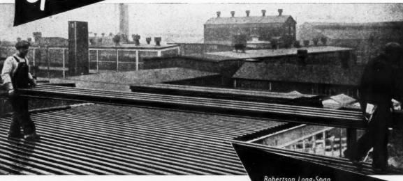
ROBERTSON Long-Span Q-Deck assures economic construction when building design takes into account the outstanding advantages offered. Centres of support may be as much as 22' 0" (the maximum length of Long-Span Deck).
