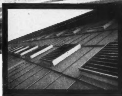
The problem of overcoming intense radiant heat in Rolling Mills has been effectively solved by employing Clear Opening Ventilators as shown inset for a number of leading Companies in the Steel Industry such as:—
