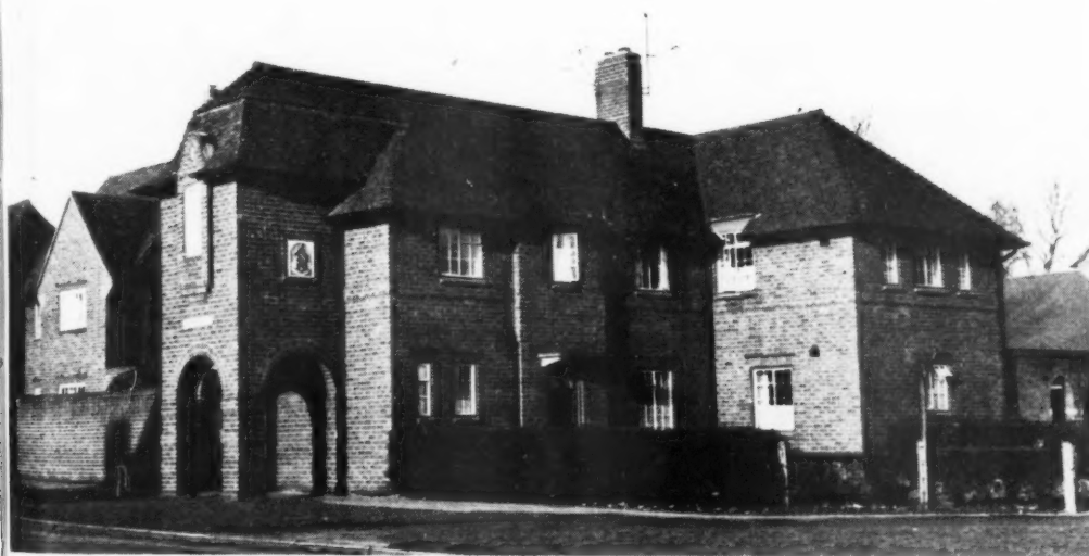
Main Entrance Feature to Shelthorpe Housing Scheme for Loughborough Corporation. Built with Tuckers "Multiruf" (Reg'd.) Facings and roofed with Tuckers Handmade Tiles. Architect: The late Barry Parker, F.R.I.B.A.
