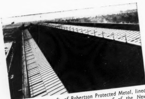
Robertson Protected Metal (lined with insulating board by the Robertson method) and Robertson Round Ventilators on the New Heavy Turbine Shop at the G.E.C. Fraser & Chalmers, Engineering Works, Erith, Kent.
