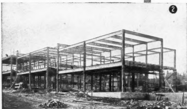
① New factory building for Messrs. William Cooke & Co. Ltd. of Rotherham. 300 ft. x 120 ft. span.
