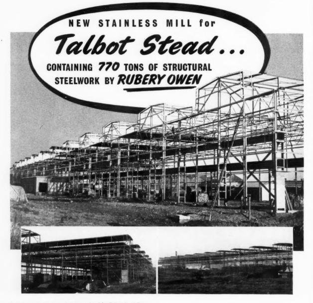
New factory building now being completed for Talbot Stead Tube Company Limited, Walsall (a T.I. Group Company) for the production of Stainless Steel Tubes. Monitor frame type structure of all-welded construction. Comprising two bays with gantry crane tracks. Each of 75ft. span and 300ft. and 660ft. long respectively. Roof and side covering and patent glazing supplied by RUBERY OWEN.
