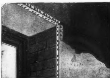
Protection of a window reveal.
