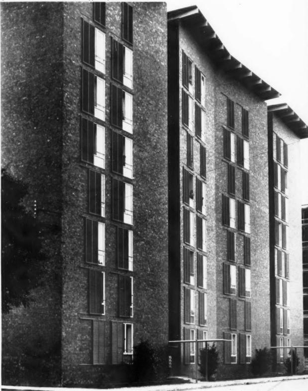
The walls are clay block with r.c. reinforcement, faced with clinker tiles—not brick. The design is interesting as a successful paraphrasing of traditional form in an industrialised architecture. Note the attic windows under the eaves.
