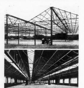
This new method overcomes the problems created when roof spans exceed 60 feet.
