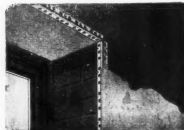
Protection of a window reveal.
