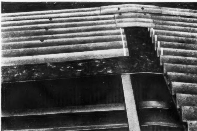
Showing the use of 1" glassfibre infill for improved thermal insulation. The flat inner linings present a clean and attractive internal finish.
