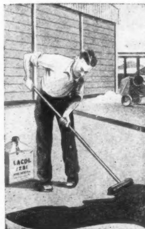
LACOL 1281 is applied cold, by squeegee or soft broom.
