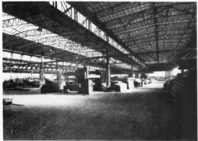
Typical example of Hills Dry Building System as applied to Factory Construction.
