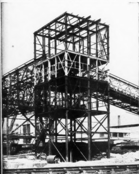
Steelwork for Raw Materials Handling Plant, installed by Mitchell Engineering Ltd., at the gigantic new Works of the Steel Company of Wales at Margam.
