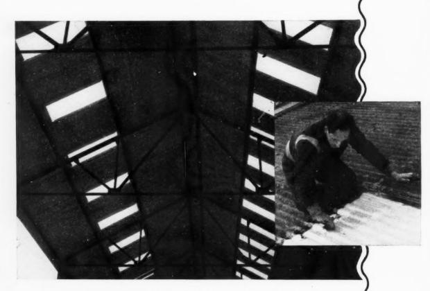
IT IS PLEASANTER and easier to work in a building that has Saropane sheets transmitting even, shadowless light. These corrugated translucent fibre-glass sheets are now made with a resin, providing even greater durability, and weight for weight they are stronger than steel.
