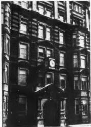
New purpose-made windows fitted into the existing wood sub-frames provide better lighting conditions and more easily controlled ventilation in Pitman's College, Southampton Row, W.C.I.—without detracting from the sturdy Victorian character of the building. ARCHITECT: T. F. A. Manning, B.A. (Arch.), A.R.I.B.A.
