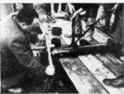
A special hand lathe is used for cutting joints on short lengths.
