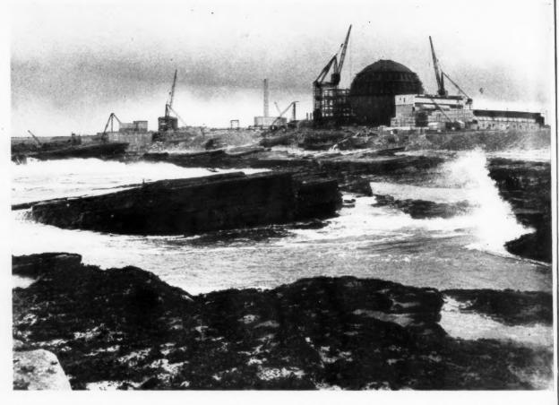
Above: Dounreay works from the seaward side, which provides one of the most dramatic views of the steel sphere enclosing the fast-breeder reactor. On the extreme left is the sea-water pump house which will
