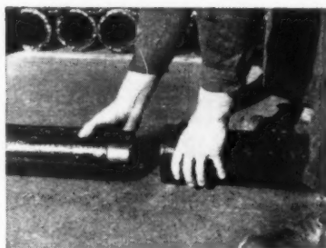
The precision-machined taper joints require no mortar or jointing compounds.
