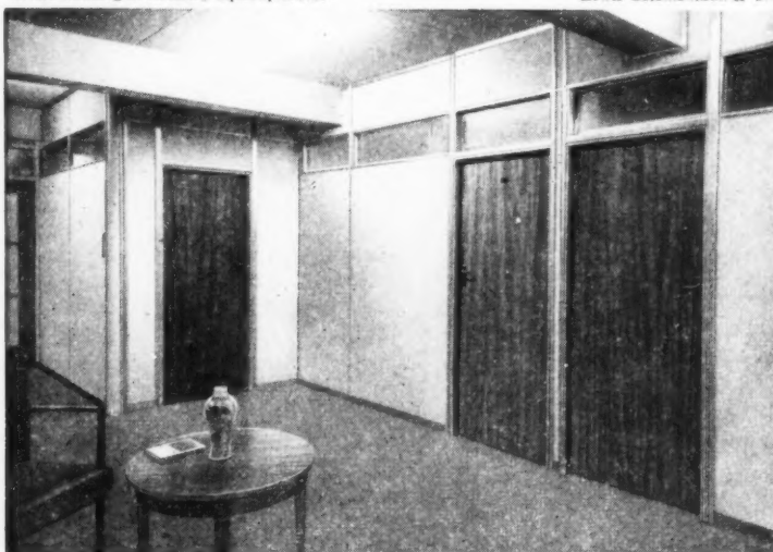
Dry construction demountable office partitions in new building in Finsbury Square, E.C.2.
