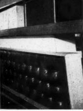
usually corrosive atmosphere, but so far they have not been painted, and although the windows were specially lacquered to maintain them in a bright condition they have had to be cleaned regularly at an annual cost not very different from the cost of cleaning the glazing itself. By contrast the lacquered aluminium inside has remained in a good condition without attention
