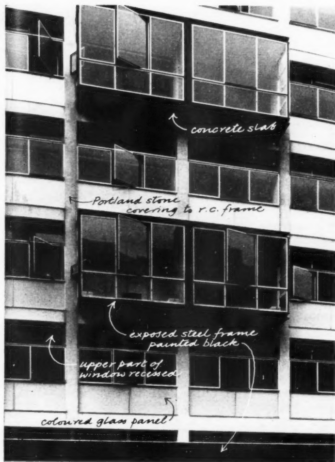
Above, central part of facade showing materials used.
