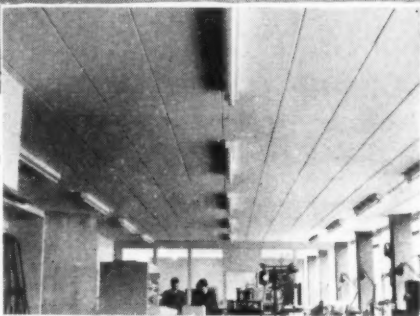
At the new Research Centre of Ruston & Hornsby Ltd., one of the most modern and well equipped buildings of its type in Europe Newalls have carried out to the order of Wm. Moss & Sons, Builders, Loughborough, Leics., the noise reduction treatment to the ceilings of the ground and first floors, using their well-known sound absorbing "Paxtiles" (Regd. Brand). The area of treatment amounts to over 1 000 square yards.
