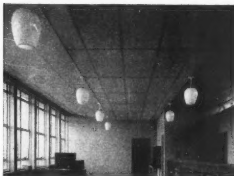
HATFIELD TECHNICAL COLLEGE Tentest Rabbit Warren Acoustic Panels, fixed with aluminium strip.
