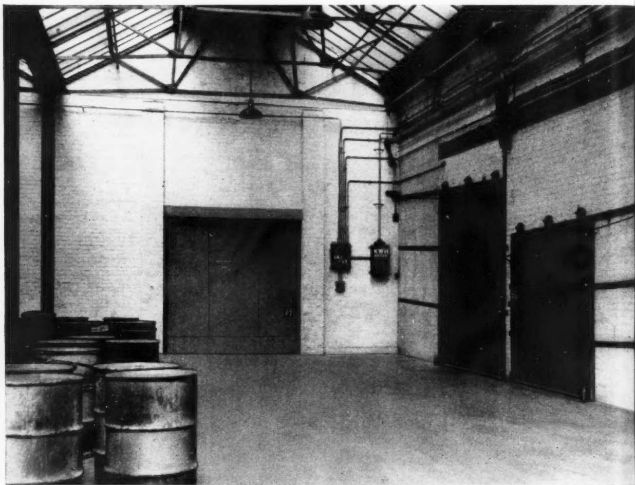
Automatic sliding composite fire doors at a reclaimed-rubber works in the North of England.
