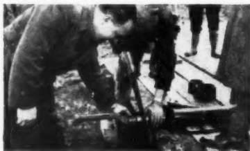
Short lengths of pipe can be cut with a coarse toothed handsaw.
