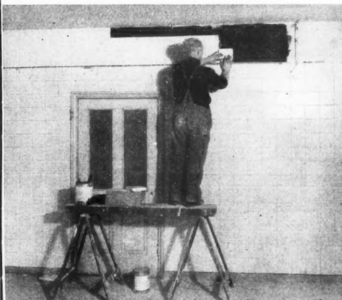
2 FIX THE TILES IN POSITION
