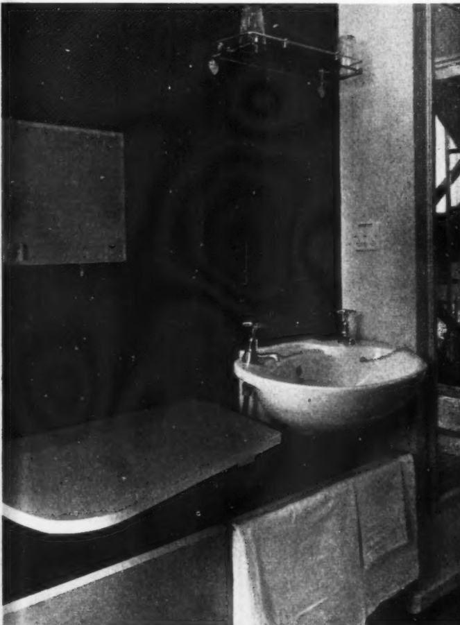
Below: the wall behind the lavatory basin is papered. A plastic-topped shelf is fixed over a convector heater, and a panel below the shelf and the basin conceals the plumbing as well as the heater unit. A universal electric shaving point is provided by the basin.
