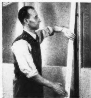
8 Pilasters are clipped on to the notches of the link plates to finish off the joints between units.
