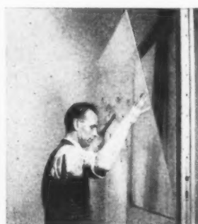
11 Any type of 32 oz. glass slips into the opening, followed by the second set of four glazing beads.
