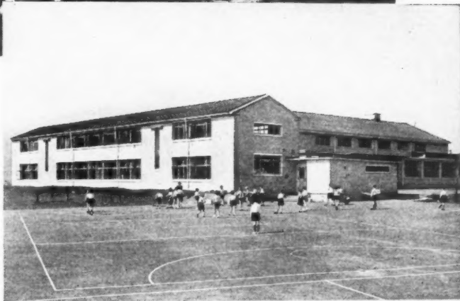
TOPHILL JUNIOR SCHOOL, PORTLAND, DORSET. Architect: J. HURST, A.R.I.B.A., Dorset County Architect. Broderick Insulated Copper Roofing at 22\frac{1}{2}^\circ pitch using 28 s.w.g. copper with special fixing to 2" Stramit.
