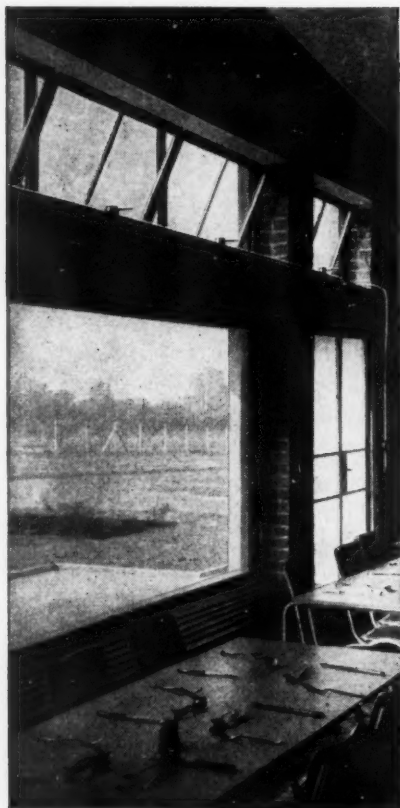
Illustration shows part of the canteen at the Administration and Design Office of W. J. Fraser & Co. Ltd., at Harold Hill, where Teleflex Remote Controls were used for window operation.
