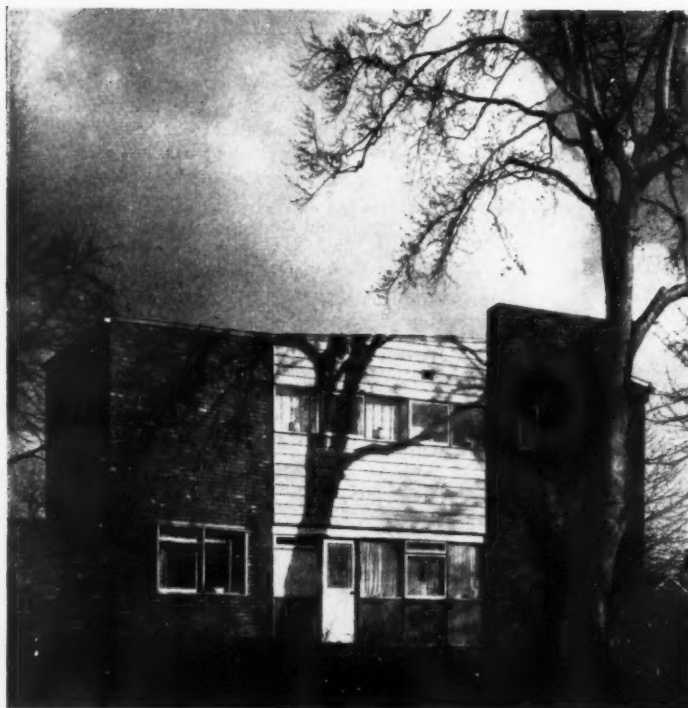
Viewpoint 10. The caretaker's house from the south-west. 11-in. cavity construction of facing brick and breeze plastered. Horizontal boards are \frac{3}{4} -in. meranti on \frac{1}{4} -in. exterior quality ply on \frac{3}{4} -in. battens on building paper on 9-in. common brick plastered internally.
