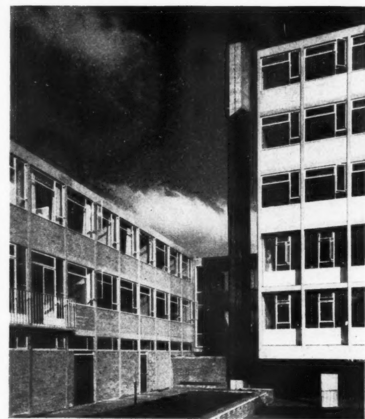
Viewpoint 4. Left, 3-storey administration block; right, classroom block. The brick-faced horizontal flue leader connects with the base of the in situ r.c. hexagonal flue, which is 6 ft. 10 in. \times 4 ft. 4 in. \times 70 ft. high. The top 3 ft. is painted with bitumen. Infill panels to administration block are of red facing brick to match the existing school and act as a foil to the teaching block, on which lower spandrel panels are lemon yellow (Archchrome 15) and upper ones are warm coloured exposed aggregate p.c. concrete.
