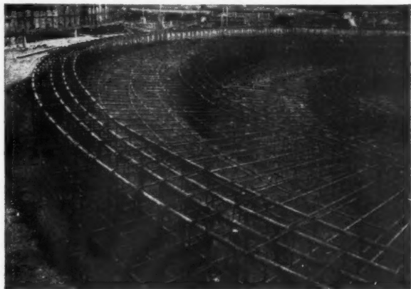
CIRCULAR BEAMS for Sedimentation Tanks at Hereford Sewage Works.
