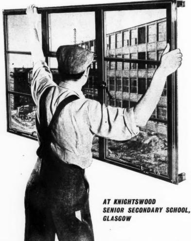
Maclean's setal Win lows are more than units which are convenient and easy to install. They make the most of the rather limited bright weather of these islands, are electro galvanised, plus two coats of paint, each stoved on separately, to offer maximum protection against wind and rain, and are as sound in body as they are delightful in use. Windows in fact that give a good name to whoever uses them. The Hamilton factory is equipped to handle the largest contracts in the shortest possible time.
