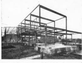
Fig. 2 (left), 4-ft. deep cellular reinforced concrete raft foundation for school on subsidence site in Yorkshire. Fig. 3 (above), Nottinghamshire school showing deep concrete foundations of former attempts to combat mining subsidence.
