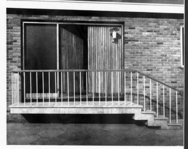
An "informal" door designed to read as a single unit with an adjacent solid panel. This has been realized by the use of teak slats. These have been fixed flush with the outside face and the side stiles have been rebated to simulate slats. To reinforce the effect of the pattern the rebates between slats have been stained matt black.
