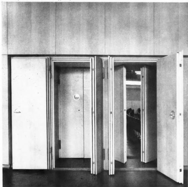
An unusual feature of these acoustic doors is that both door frames and jambs are formed in mild steel angles. All doors are double-rebated (including the thresholds), the metal parts which enclose the mineral wool core are screwed together with felt seatings between and rubber sealing strips are glued to the re-entrant angles of the door rebates to ensure silent closing.
