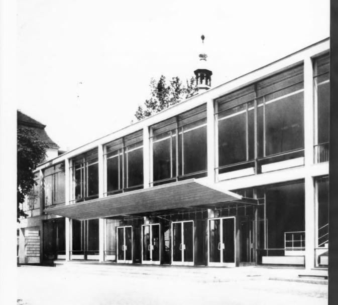
This is a good example of a type of canopy which is cranked in section, with patent glazing on the surface adjacent to the facade and zinc cladding on a steel and timber frame on the surface farthest from the facade. Both surfaces discharge into a central gutter from which water is conveyed inwards to the building face by a single pipe which continues in the line of the outer slope. The horizontal ribbing on the underside is formed by the zinc welts.
