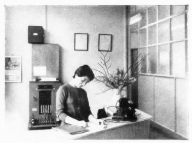
The smart appearance of the office of Max Rayner (Artwork) Ltd. owes much to its new, glazed Stramit partitions in I-in. x 4-in. timber framing: the Stramit is held in position by quadrant moulds.
