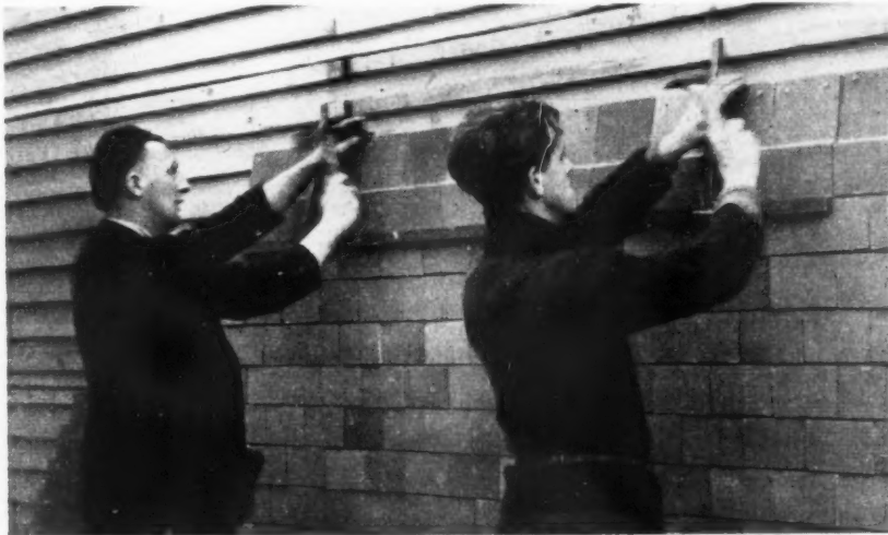
Keytoclad tiles being hung.
