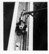
3-way fixing - but in this case they are finally bolted in for extra strength
