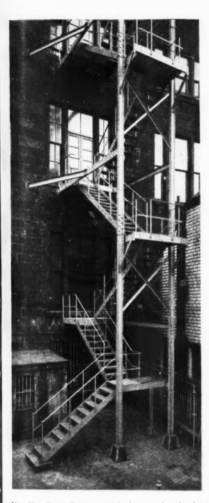
Lion Fire Escape Stairs are made for strength and safety Available either straight or spiral, they are constructed in steel with cast iron perforated treads and landing. For over sixty years Lion Foundry Co. Ltd. have been supplying and erecting fire-escape stairs for Government Buildings, Local Authorities, Hospitals, Office Blocks, Theatres, etc.
