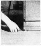
unit of partitioning are screwed bolted to the sole plates. All units drop into ready pressed out pockets are interchangeable.
