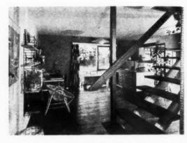
Above: the eastern half of the ground floor studio. Below: the dining area seen from the studio. The free standing staircase has hardwood treads, carried on mild steel channels. Left: the western half of the studio. The cupboard units and handrail at first floor level are at the open end of the gallery.
