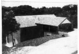
Two similar staff houses were required by the Housing Trust of the Federation of Malaya, one (illustrated in these pages) for their chief architect and one for their chief engineer. Owing to the steep slope of the site, accommodation was designed on four levels, with access at the highest level and bedrooms on the lowest level. Only two bedrooms were required, due to the practice of sending children back to the U.K. for their education, at an early age.
