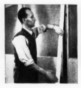
8 Pilasters are clipped on to the finish off the joins between units.
