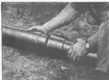
The precision-machined taper joints require no mortar or jointing compounds.
