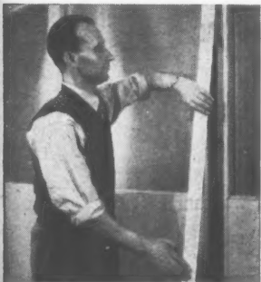
8 Pilasters are clipped on to the notches of the link plates to finish off the joins between units.
