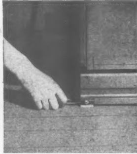
2 The 40" wide, modular units are bolted to the sole plates. All units are interchangeable.
