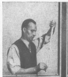
10 Four rubber-buffered glazing beads clip in. Special beads are available for double glazing.
