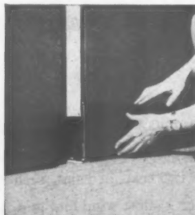
9 Skirting is clipped on to the bottom of each unit. Plinths cover the joins in between.
