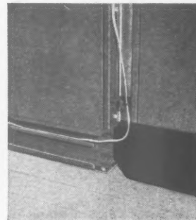
6 Electric wiring runs down between partitioning units and along specially provided channels at the bottom.
