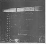
The Udall Lintol, having bee stressed, is now ready to tak the full load of the brickwor structure above. Th and opening is then cut away
