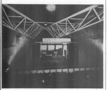
The auditorium roof is supported on welded-tube steel space frames, supported on the brick piers at the foyer end, and on the proscenium wall at the other. The precast ceiling slabs are painted matt black, and the space frames butter yellow. All the curtains are drawn back, including the side entrances. The cleaners' lights are swung out into position from the side spot boxes.
