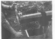
A special hand lathe is used for cutting joints on short lengths.
