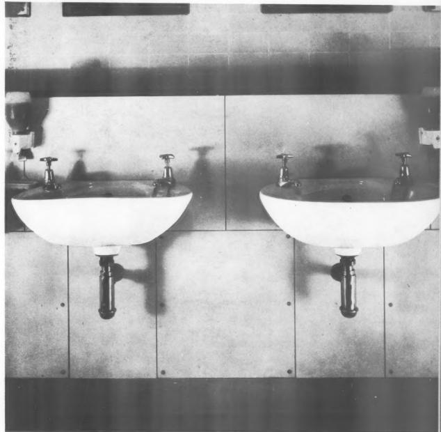
The main point of technical interest about these washbasins is the substitution of a clamp for the usual bracket. The panels on which the basins are fixed are of melaminefaced sheet glued to timber framing, the lower panels between the basins being fixed with cups and screws to give access to the pipework behind.
