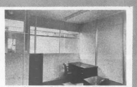
Section of Estimating Office : Half-glazed and full-height partition constructed with Conpactite and Tricore panels in aluminium framing
