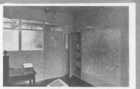
Corner of Wages Office : Half-glazed Glinex partitions with polished timber framing and Compactom built-in cupboards.
