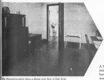
For new or replacement floors. Hardwood Strip is fixed to the ordinary joists by means of hidden nailing.
