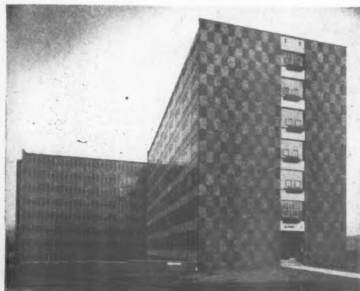
Viewpoint 7: a general view of the building from Dartmouth Street. Flank walls are clad with pre-cast concrete blocks with two different colours of exposed aggregate finish. Each block, approximate size 2 ft. 6 in. x 3 ft. 6 in. x 3 in., is held back to the building with two copper ties which are grouted in. Edge panels are specials with a change in direction of 90 degrees to meet the curtain walling on the centre line of the last column.
