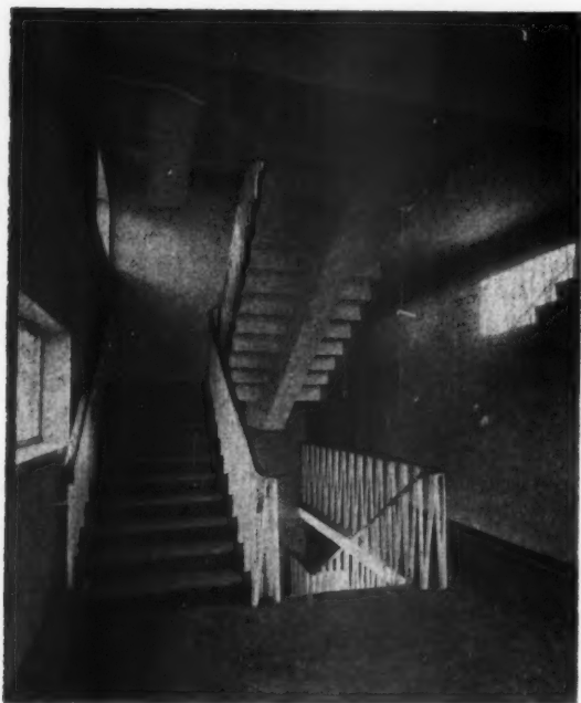
Detail of an emergency escape stair, which also serves as a subsidiary entrance. The door on the right hand side of the landing leads directly into a workspace. The whole of the staircase is reinforced concrete left fair-faced and the result is a strong, clean structure which combines not too happily with the diagonal m.s. balustrading. The finish to the treads is a red granolithic with a non-slip tile nosing.
