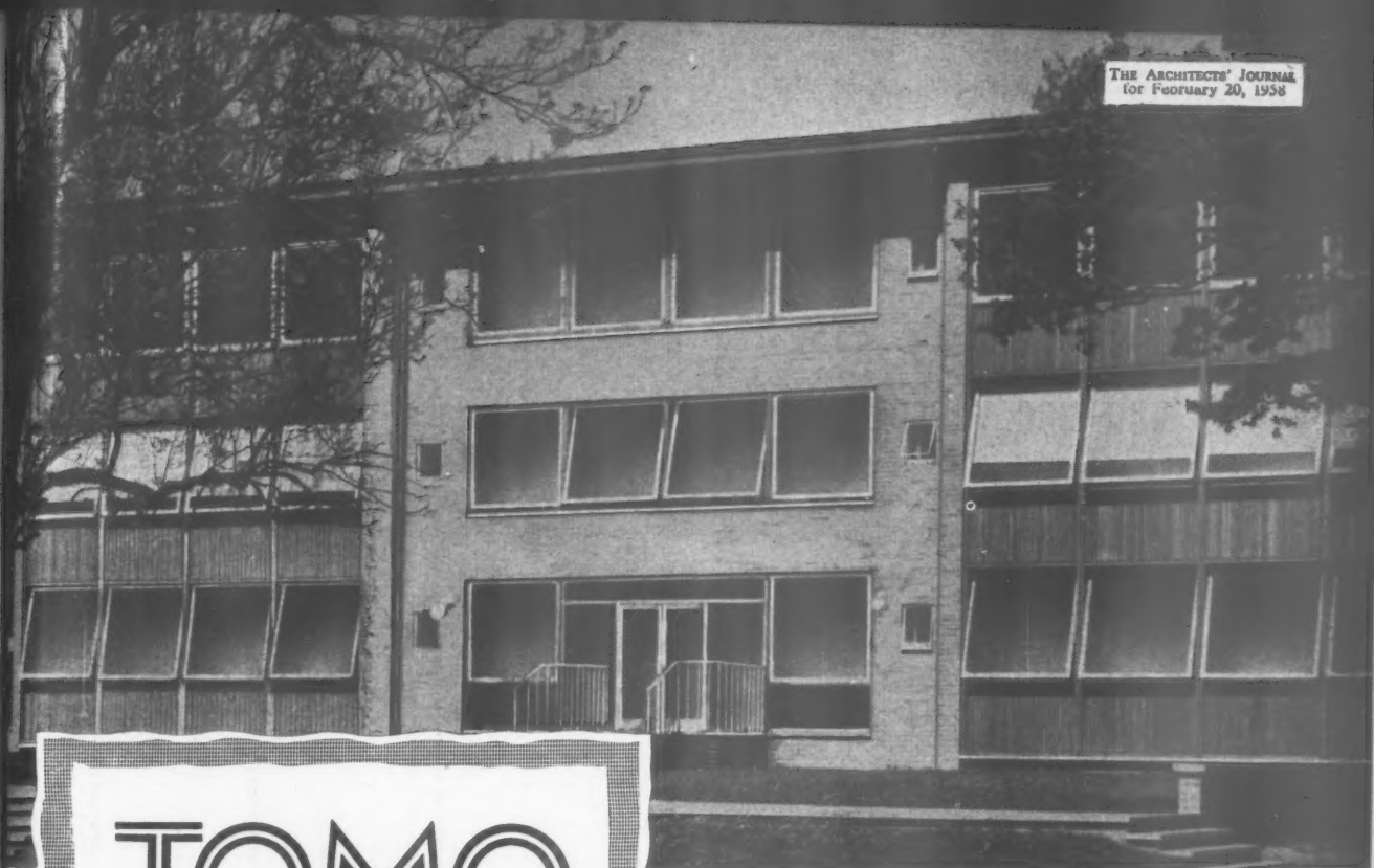
Horizontal-pivot-hung TOMO WINDOWS are incorporated in the attractive and economical curtain-wall at the Bishop Simpson Secondary School. Architect: Charles H. Pike, F.R.I.B.A.
