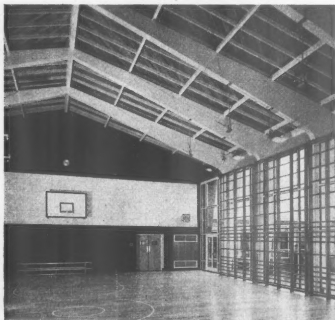
Photo shows 'WOODWELD' Portal Frames supplied for the Quarrendon Secondary Modern School, Aylesbury. These Portals carry light Gymnasium equipment in addition to Roof. Span 47 ft. 6 ins.
