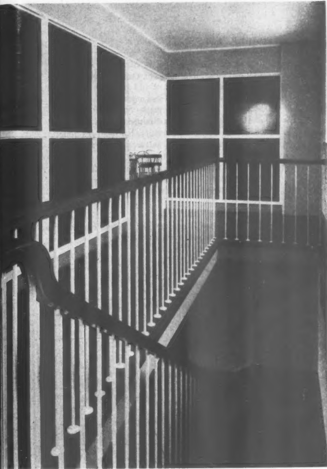
The staircase and first floor landing. 2-in. hardwood treads are carried by a r.c. stringer beam and there are no risers. The handrail is 2-in. x 3-in. hardwood.
