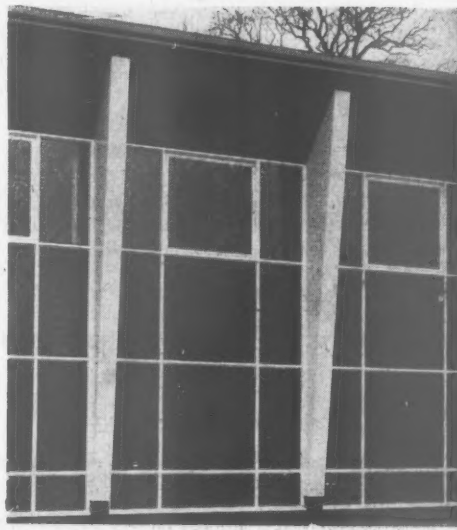
Photo shows 'WOODWELD' Portal Frames supplied for the Quarrendon Secondary Modern School, Aylesbury. These Portals carry light Gymnasium equipment in addition to Roof. Span 47 ft. 6 ins.
