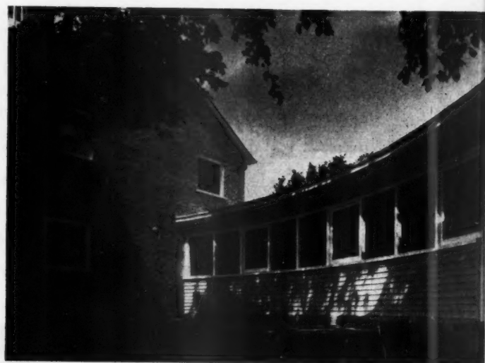
Viewpoint 3: the single-storey changing room wing, which is faced, on this elevation, with 6-in. \times \frac{3}{4} -in. horizontal weatherboarding on timber studs at 2-ft. centres.
