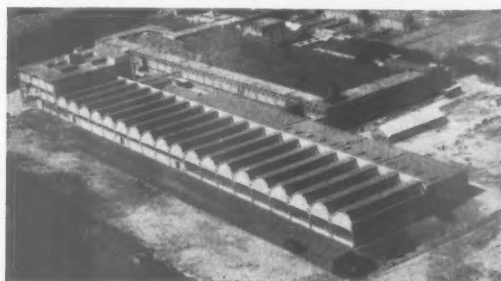
2 North light glazing at Scribbans-Kemp Bakeries Ltd., Grimby. Architects: William Saunders & Partners. Partner-in-charge: B. G. Gibson, L.R.I.B.A.
