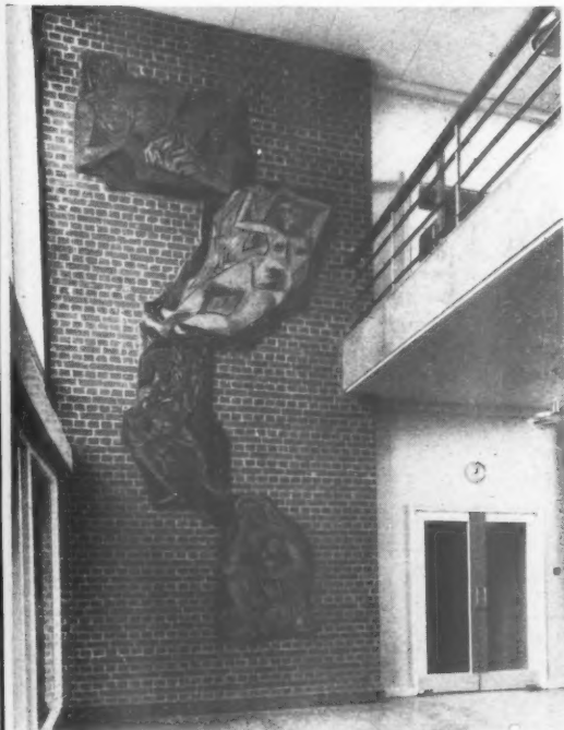
A detail of the sgraffito mural panels, by John Sutton, appearing on a blank wall within the entrance hall. This involves a technique of etching plaster to expose colours applied in superimposed coats. The bronze balustrading to the first floor landing can also be seen; the Derbydene stone on the edge of the landing is also used as a facing to the staircase in this hall.
