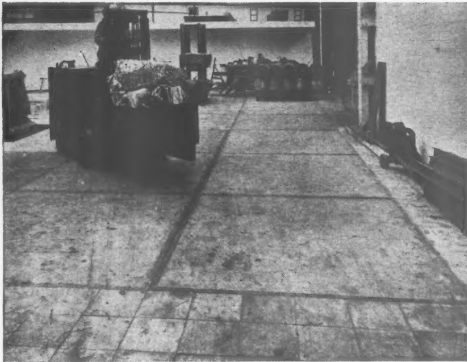
The illustration shows Stelcon Raft flooring laid at the Carver Street Works of D. F. Tayler & Co. Ltd. Birmingham.
