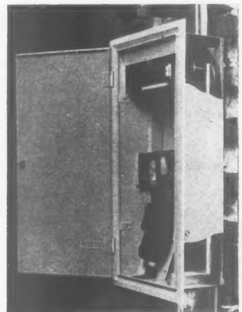
Fig. 5 (above), consumer's supply control unit.
