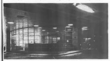
On the right is the ramp up to the first floor. Cars arriving in the basement can either pass over the inspection pit (on the left of the photo below) or by-pass it, going through to the parking and washdown area beyond. analysis
