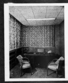
Director's office: Insulated double-wall Compactite partition, veneered and polished light oak. Fitments designed and constructed by Compactom. Acoustic tile ceiling with flush lighting.
