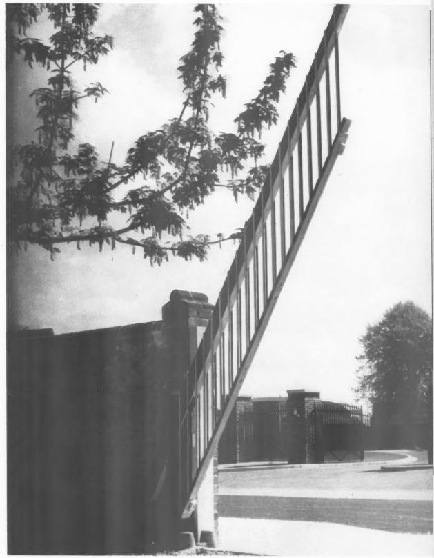
This gate closes n wide opening with n single leaf which is easy to open and, as it does not exert eccentric pressure on post or hinge, will not sag. The width of the opening is about 12 ft. The gate itself (i.e., all on the opening side of the point of balance) weighs about 252 lb., but as this is exactly balanced by the counterweight there is no weight to lift. The twin bollards are to prevent the lower rail from swinging when the gate is lowered.
