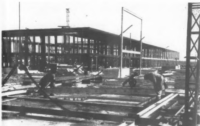
Fig. 12, two-storey site-welded frames at secondary school, Hunstanton. Architects: Alison and Peter Smithson. Consulting engineers: Ove Arup & Partners.
