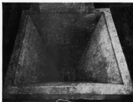
Completed pit surrounded by 9' 6" head of subsoil water.
