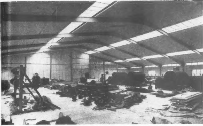
Fig. 3, a portal frame in a spinning mill at Witney, Oxon. Architects: Fielding Dodd and Stevens. Engineers: Conder Engineering Co. Ltd. This and all succeeding photographic examples were designed by plastic theory.
