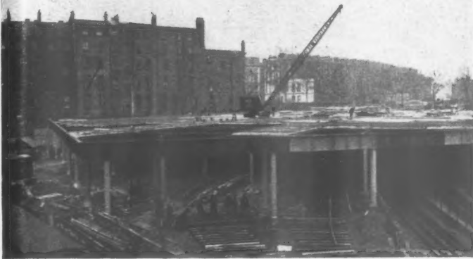
Fig. 7, welded main girders and stanchions at West London Air Terminal. Engineer: C. E. Dunton, Chief Engineer to London Transport Executive.
