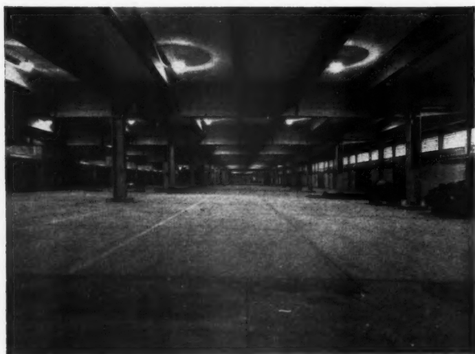
Fig. 5, a welded plate girder floor system for heavy loading in Transit Shed No. 102 at Southampton. Consulting Engineers: Scott & Wilson, Kirkpatrick & Partners in collaboration with the Docks Engineer, J. H. Jellett. Photo by courtesy of the British Transport Commission.
