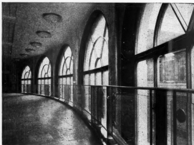
Above: Main glazing, incorporating 'Insulight' Double Glazing Units. Balustrade panelled with flat and bent \frac{1}{4} " Polished Plate Glass.
