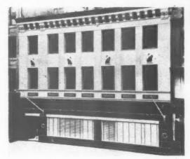
There need be nothing stereotyped about SEAPORCEL frontages. The panels for each separate job are designed and enamelled in pattern, style and colour to the architect's specification.
