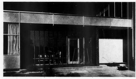
Viewpoint 3: detail of the main entrance. The external cladding: aluminium droppers support asbestos panels (with woodwool core) painted red (Archrome 4) below the window and light grey (9.099)
