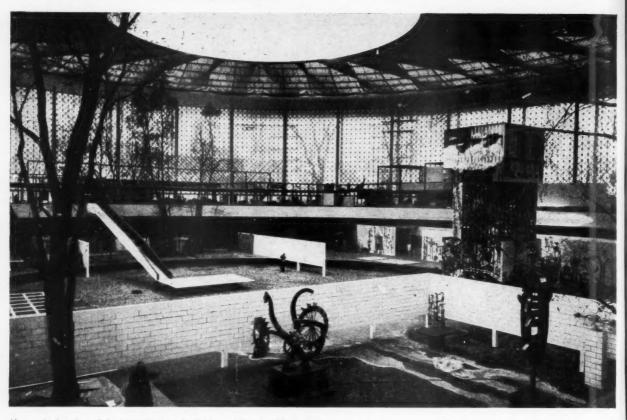
Above, the interior of the hypaethral main U.S. pavilion (architect, Edward Stone) showing the steel cylinder, which is suspended by cables from the eaves to form the roof. Mannequins parade continuously down the ramp to the platform standing in the central pool of water. Below, the less sophisticated Russian pavilion. More pictures are on page 601.
