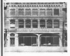
These 'BEFORE-AND-AFTER' pictures, taken twenty-two years ago, show how effectively SEAPORCEL PANELS can be used to modernize old-fashioned frontages without demolishing existing masonry.
