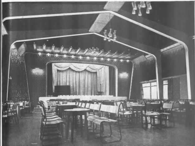
WOODWELD PORTAL FRAMES merge successfully into contemporary as well as conventional building design. Above photograph shows 36-ft. span Portal Frames used in the main hall of the Bank Hall Institute, Burnley. A Plywood beam is used over the proscenium and straight Box Beams with solid columns and Roof Trusses have been used in this structure.
