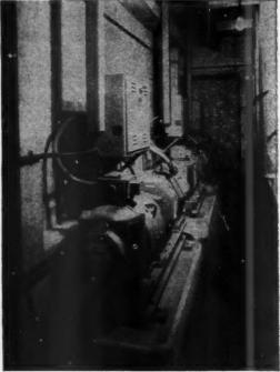
Three of the seven 21 kW motor generator sets associated with each lift installation,
