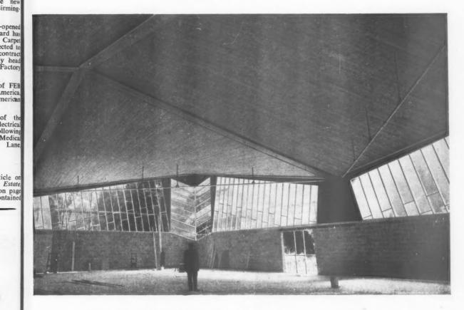
This unique example of timber roofing, has been erected for the Wilton Royal Carpet Factory. The roof consists of four timber shells, each measuring over 57 feet square.
