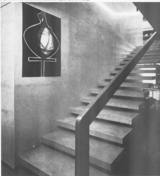
There is nothing particularly new about the cantilevered stair treads. What is of interest is the thorough manner in which the problem of the offside handrail has been faced: a Swedish pine rail, massively reinforced with steel, runs direct from the lower to the upper structural floor. The treads, on being cast into the wall, are tilted slightly upwards so that they settle to the horizontal.
