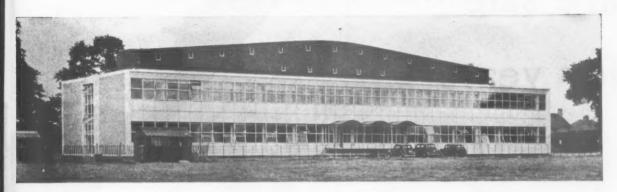
Alphamin Sandwich has been used extensively for wall cladding at the Ministry of Agriculture, Fisheries and Food new Biological Products and Standards Laboratory at Weybridge. The sandwich was developed by Alphamin Ltd in collaboration with British Aluminium, and consists of a 1" pure baked cork slab bonded between 22 s.w.g. aluminium sheets.
