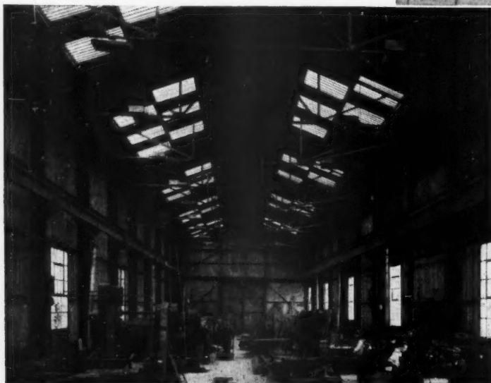
Corrugated 'Perspex' roof lighting installed in the works of Mitchell, Russell & Co., Bonnybridge. Photographs by arrangement with Newton, Robertson & Co. Ltd., Glasgow.
