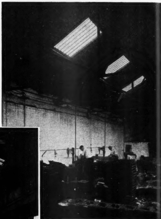
Corrugated 'Perspex' roof lighting installed in the works of Mitchell, Russell & Co., Bonnybridge. Photographs by arrangement with Newton, Robertson & Co. Ltd., Glasgow.
