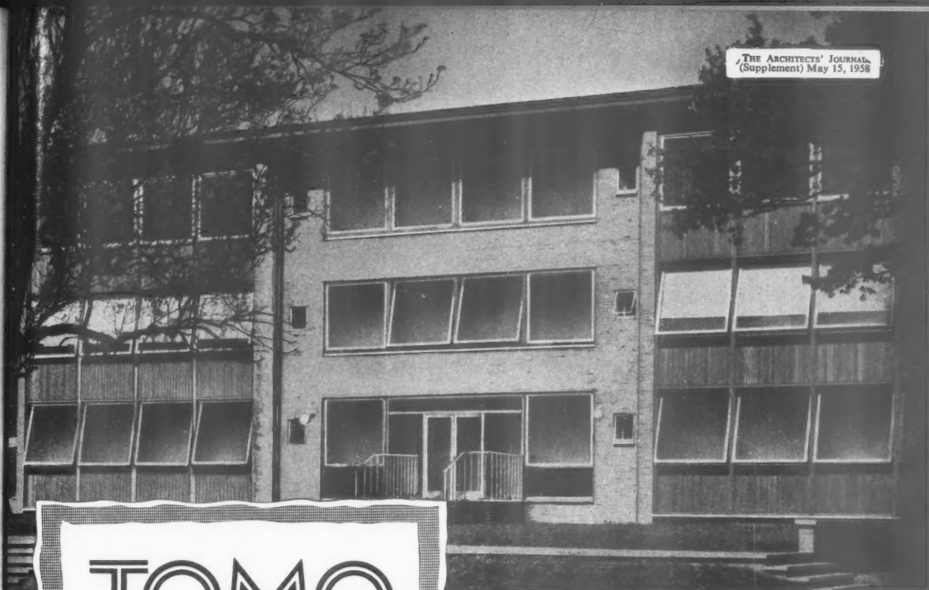
Horizontal-pivot-hung TOMO WINDOWS are incorporated in the attractive and economical curtain-wall at the Bishop Simpson Secondary School.
