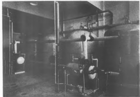
4,160 gallons storage of hot water with 6 hour recuperation under thermostatic control at 150°F.
