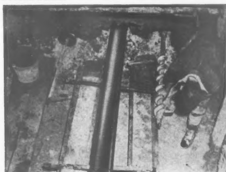
A 6" bore Temple Tube drain for chrome acid effluent, 20 ft. under the production assembly line, being installed (through thrust bore holes) at Messrs. Vauxhall Motors Ltd., Luton. An air test of 2½ p.s.i. held for 20 minutes was immediately applied and found satisfactory. The material was tested in Messrs. Vauxhalls own laboratories for acid resistance.
