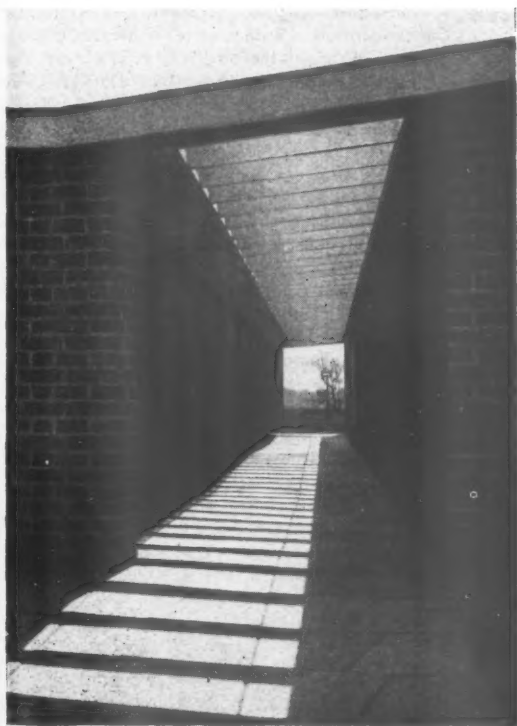
The last photograph shows the cycle shed (viewpoint 5) which has a timber joisted roof, the centre portion forming a pergola.
