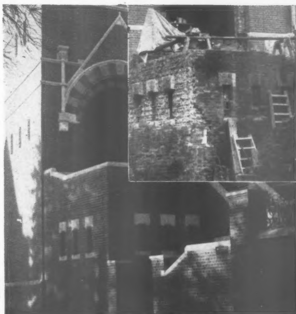
Part of the completed building. The inset photograph shows: right, the ruinous condition of the old brickwork and left, work cut back ready for resurfacing.
