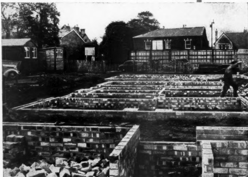
'Phorpres' Fletttons being laid in foundations of the Birmingham Corporation Housing Development at Laurel Road, Handsworth, Birmingham
