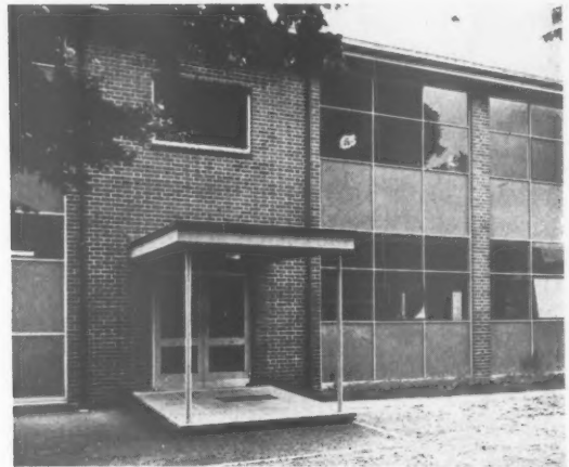
Two views of the science block at Magdalen College School. Below, the south-west elevation. The structure consists of blue Stafford piers, concrete floors and timber roof with asbestos slates. Above, the north elevation with an appropriately simple but generous canopy over the entrance.
