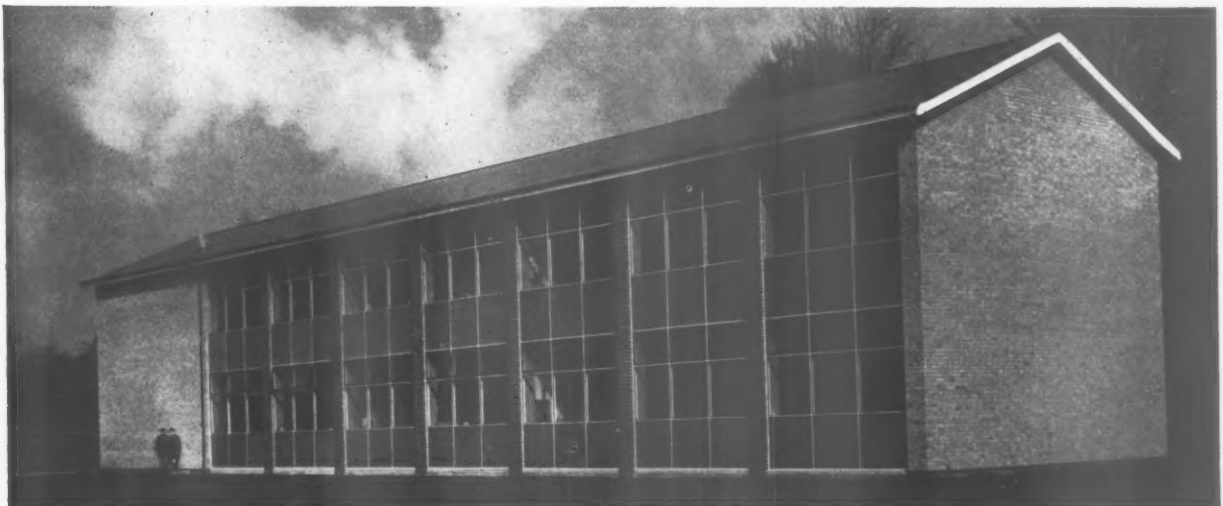
Two views of the science block at Magdalen College School. Below, the south-west elevation. The structure consists of blue Stafford piers, concrete floors and timber roof with asbestos slates. Above, the north elevation with an appropriately simple but generous canopy over the entrance.
